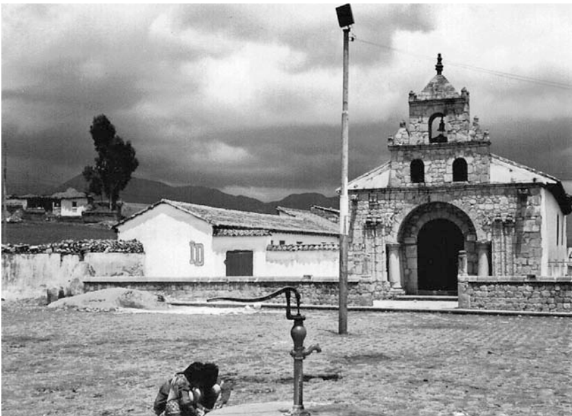
FIGURE 4. Church of Balbanera, by Lake Colta, built by Spaniards in 1534
