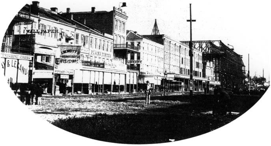
CANAL STREET IN THE 1850S. (NOTE THE STORE ADVERTISING “PIANO FORTES.”)
