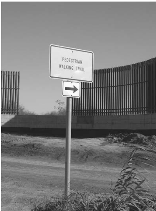
Figure 11.1 Construction of the border wall at Hidalgo Pumphouse and World Birding Center. Photo courtesy of Margaret E. Dorsey, 2009.
