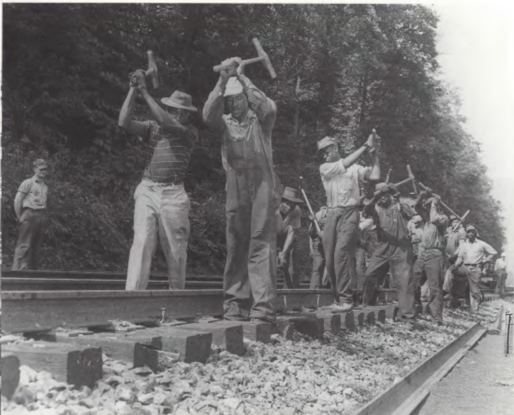
Chesapeake & Ohio trackmen spiking down a new rail, 1944 (Courtesy Chesapeake & Ohio Railway)
