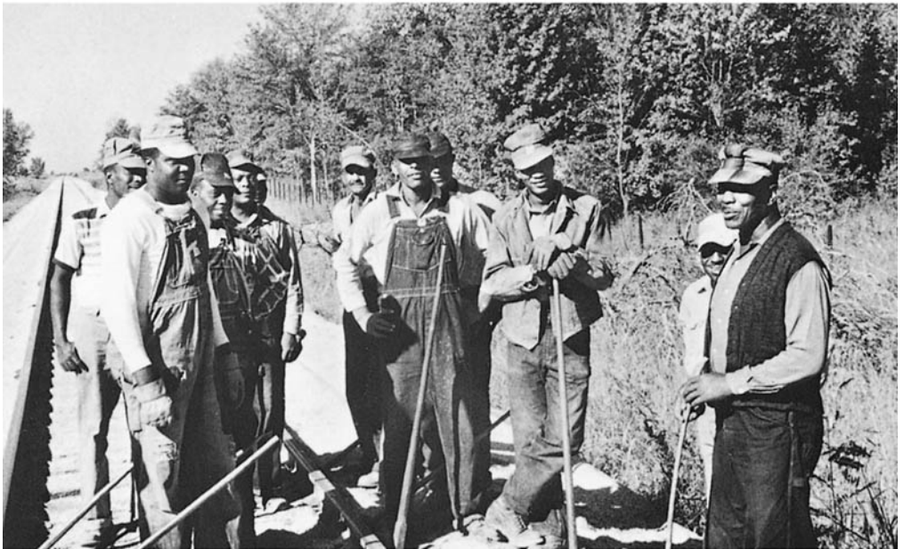
(Top) Downhome section gang with section boss (left) verifying alignment from a distance; ten section hands (center) rapping steel on steel; and section foreman:
